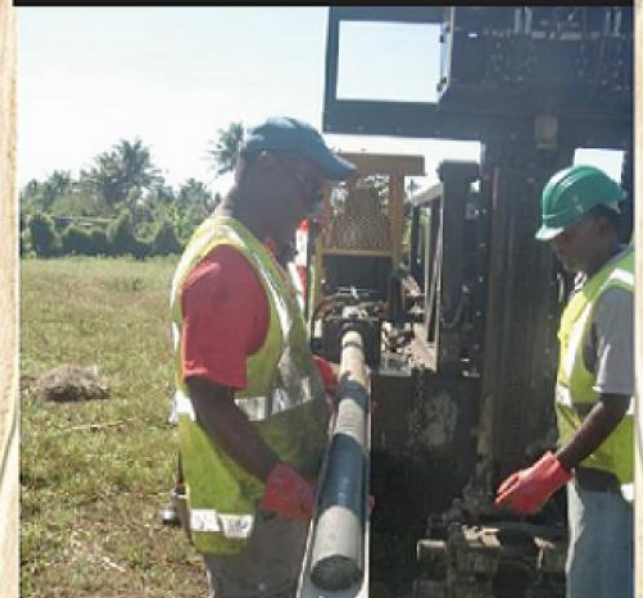
Soft sediment “core” being extruded from the sonic drill
