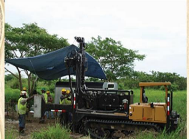
Sonic drill rig in use by Dome at Nasivi Delta
