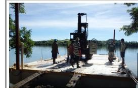
Dome's sonic drill being mounted on a barge for drilling in the Sigatoka River bed.
